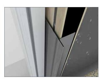
**NOTE!** If using unpainted aluminium in connection with fibre cement products, be aware of surface oxidation.
