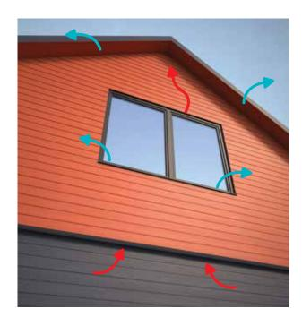
This passage must be a minimum of 10mm in the top and bottom or equal to 100mm per m<sup>2</sup>. If grids or similar are used, the openings must equal 100cm<sup>2</sup> per linear meter.
